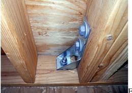
Each project is different, though at strategic points hold-down connectors may be specified, along with extra bolts, beams, metal strapping, shear walls, insert shear panels or steel plates. Your project may include any or all of the above.
