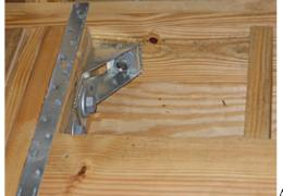
A hurricane tie is a small, but mighty piece of hardware designed to hold roof rafters to the walls of the house. There are a wide variety (whole catalogs) of clips that can be installed on any roof / rafter /wall configuration. These generally cost just a couple bucks apiece (note that hundreds may be required, depending on house size).
