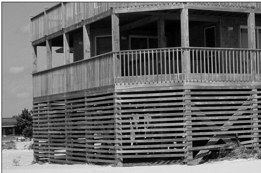
Figure 4. Wood slats installed flat against foundation pilings
